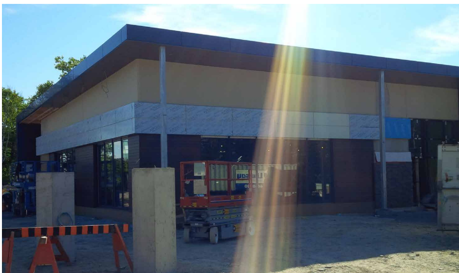
The exterior of the new NSNU building begins to take shape
