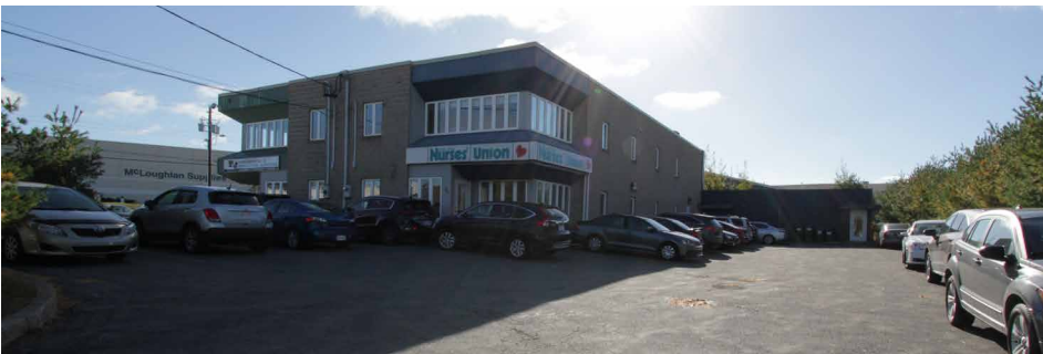
An overflowing parking lot and chronic double-parking are just some of the problems solved by a new building
